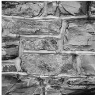
18th C. limestone, ridge pointing, lime-sand mortar
