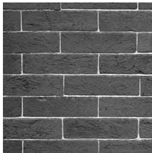
19th C. ground face brick common bond, narrow mortar joints
