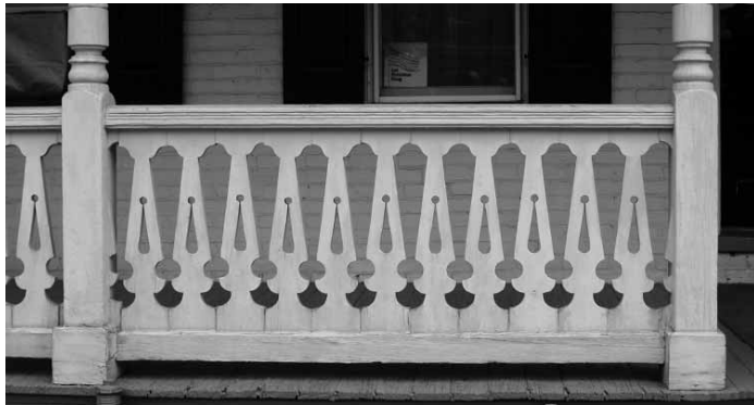
Flat bandsawn porch balusters
