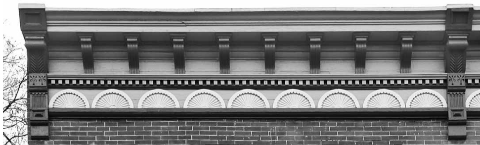
Elaborate wooden bracketed cornice and entablature
