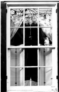
above left: Wooden window sash with individual panes of glass, held in place by muntins is the traditional and honest form of old-house window. above right: Plastic sash with fake muntins, often called "grilles" do not have the same character as the real thing.
