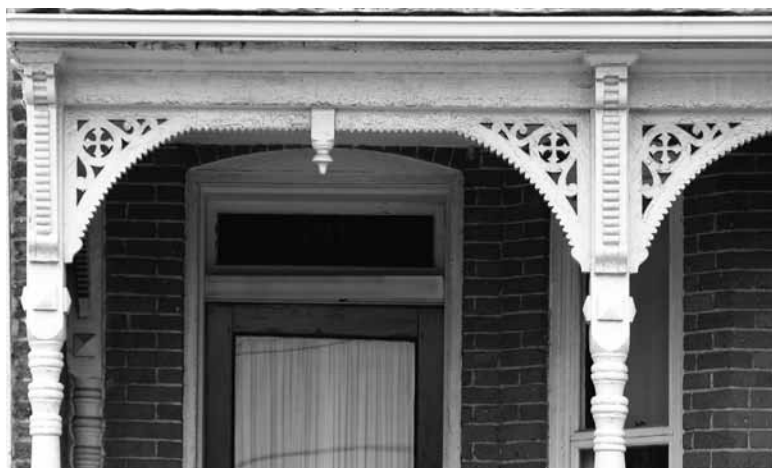
Wooden "gingerbread" braces and brackets
