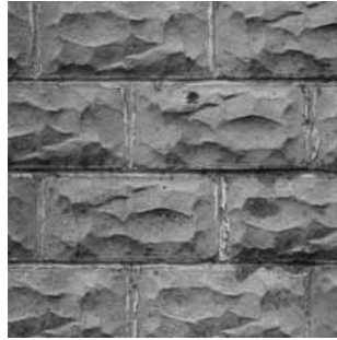
Home-made concrete block, made with a Sears Roebuck mold, an endangered material.
