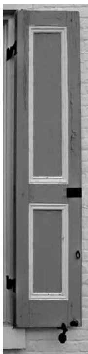
Original shutters and iron hardware
