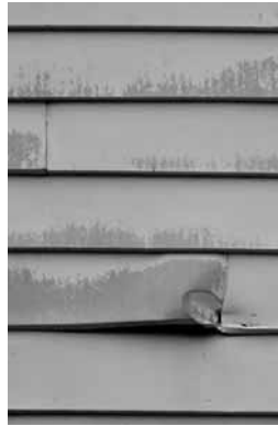
above, left: Wooden siding is a traditional building element and an honest material. above right: Aluminum siding is a poor imitation. Fiber cement board (not shown) is a much more appropriate and longer lasting substitute.
