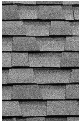
above left: Slate is a natural material. A slate roof can last hundreds of years. above right: Asphalt "architectural" shingles look nothing like slates in texture or scale and are a poor substitution. Other synthetic slates, such as recycled rubber, are a better alternative.
