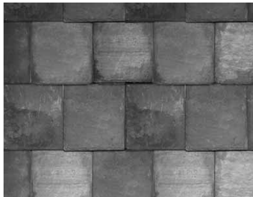
above: Slate is a natural material. A slate roof can last hundreds of years. Several modern materials can be used to replace broken slates if natural replacements are not available.
