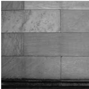
20th C. coursed ashlar cut limestone, minimal mortar joints
