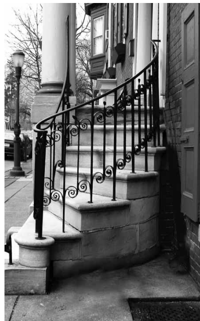
Hand-made wrought iron railing
