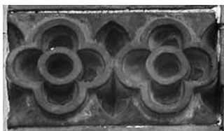
Terra-cotta trim, close-up
