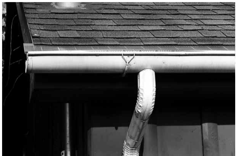
above: Half round gutter and round downspout
