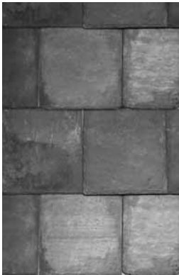
above left: Slate is a natural material. A slate roof can last hundreds of years. above right: Asphalt "architectural" shingles look nothing like slates in texture or scale and are a poor substitution. Other synthetic slates, such as recycled rubber, are a better alternative.
