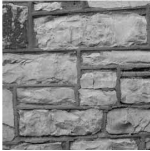
19th C. limestone, ribbon pointing, red sand mortar
