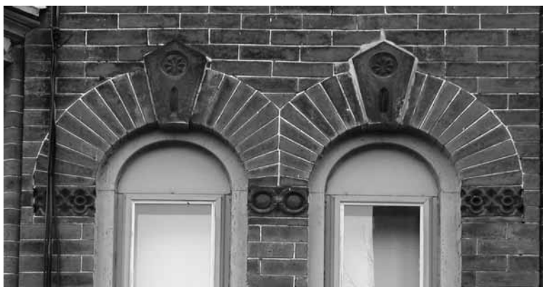
Rubbed brick arches with terra-cotta trim
