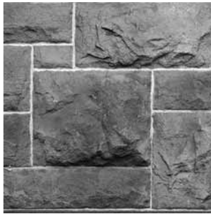
19th C. rusticated broken ashlar sandstone, flat struck mortar joints
