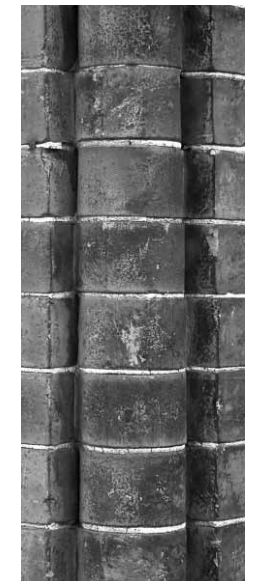
Molded brick corner
