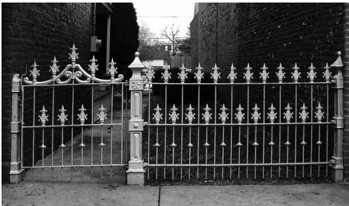
Fence and gate with cast iron posts and decorative detailing
