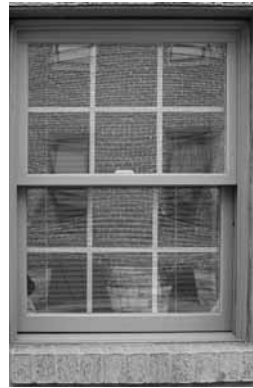
above left: Wooden window sash with individual panes of glass, held in place by muntins is the traditional and honest form of old-house window. above right: Plastic sash with fake muntins, often called "grilles" do not have the same character as the real thing.
